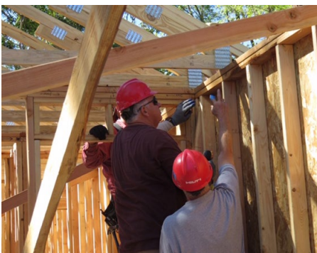
Installing trusses on new Habitat home, Oct 2019
